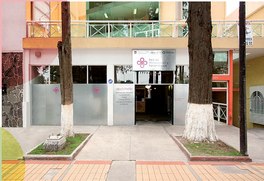
A typical façade: Toluca 2
