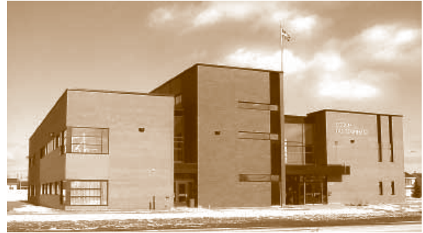
Le Tournant School, St-Constant, Quebec. The solar walls run the full height of the building on either side of the central section.
