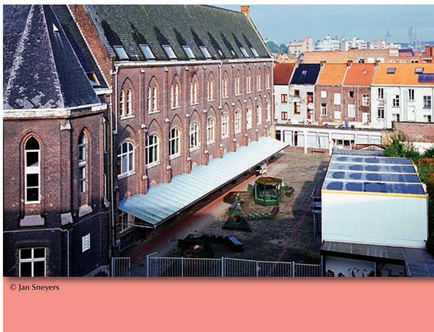
School building with temporary container classrooms
